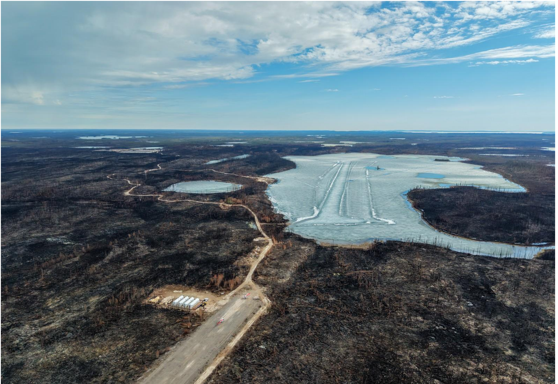
Figure 5: Nechalacho Airstrip, Fuel Storage Area, roadway to other locations and seasonal ice road for winter access.
