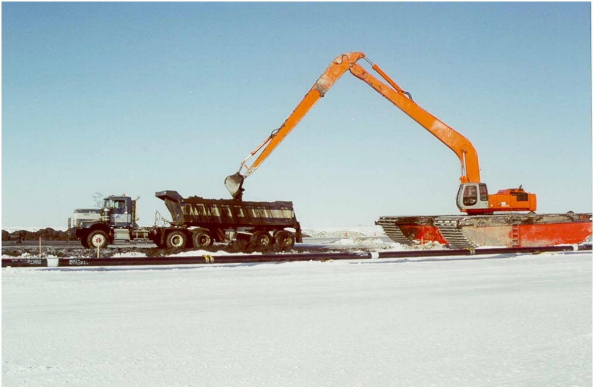
Figure 8: Trenching from the Ice using Extended Reach Backhoe
