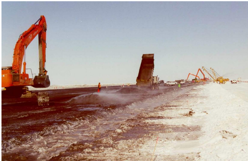
Figure 11: Backfilling of Trench
