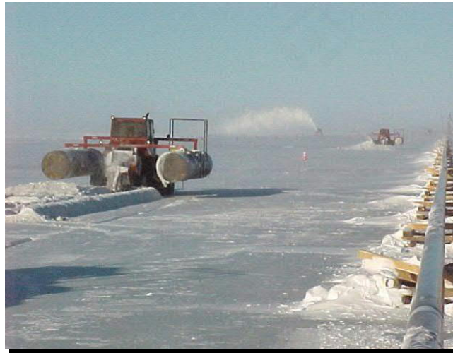
Figure 7: Cutting of the Ice using Ditch Witch Cutter
