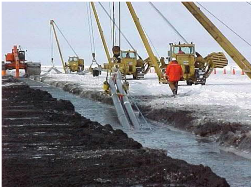
Figure 10: Lowering of Pipeline through Ice Slot into Trench
