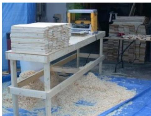
Several boards cut and planed are ready to be formed into their proper shape and marked for size
